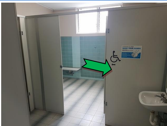
Photo 11. Interior, toilets, partition walls – non asbestos-containing fibre cement sheeting.
