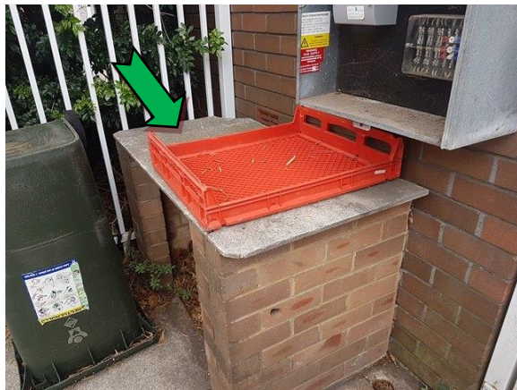
Photo 3. Exterior, south-west elevation, water main cover – non asbestos-containing fibre cement sheeting.
