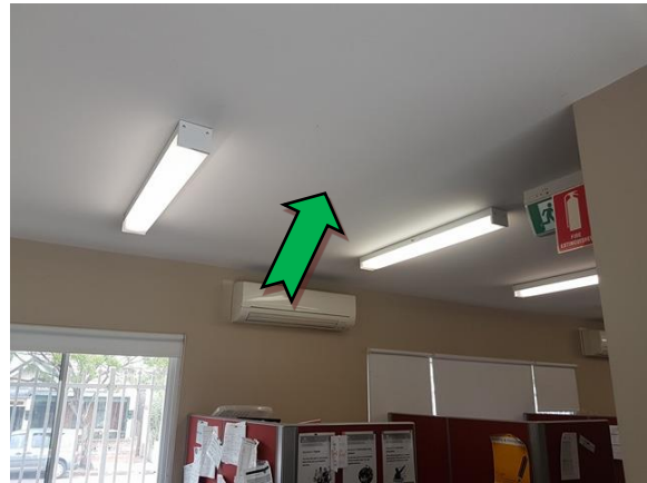
Photo 16. Interior, throughout, ceiling – white upper coloured paint system.
