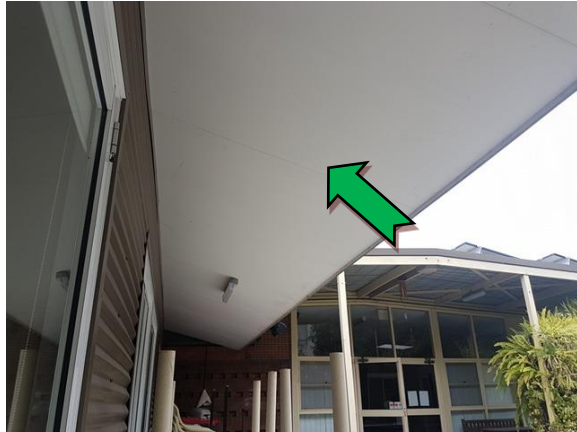
Photo 1. Exterior, north-east elevation, awning – non asbestos containing fibre cement sheeting.
