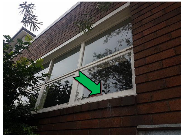
Photo 4. Exterior, south-west elevation, window frames – non asbestos-containing caulking.
