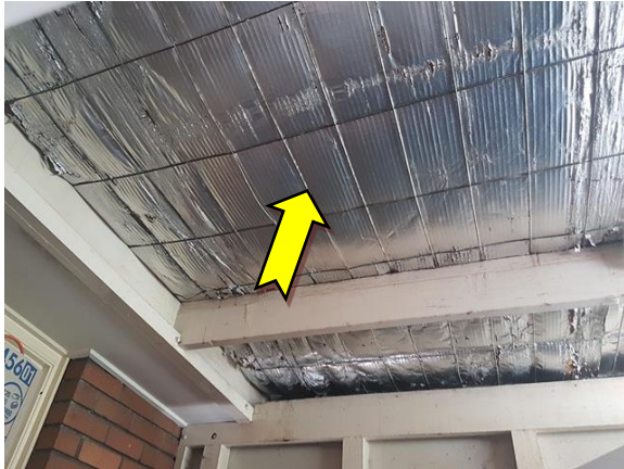
Photo 13. Interior, throughout ceiling void, sarking – suspected SMF insulation.
