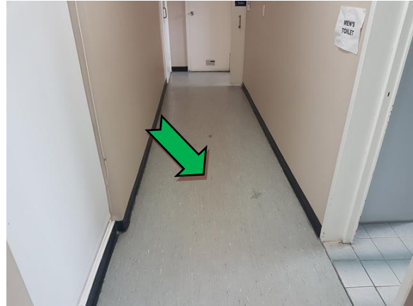
Photo 8. Interior, northern elevation, hallway, floor – non asbestos-containing sheet vinyl.
